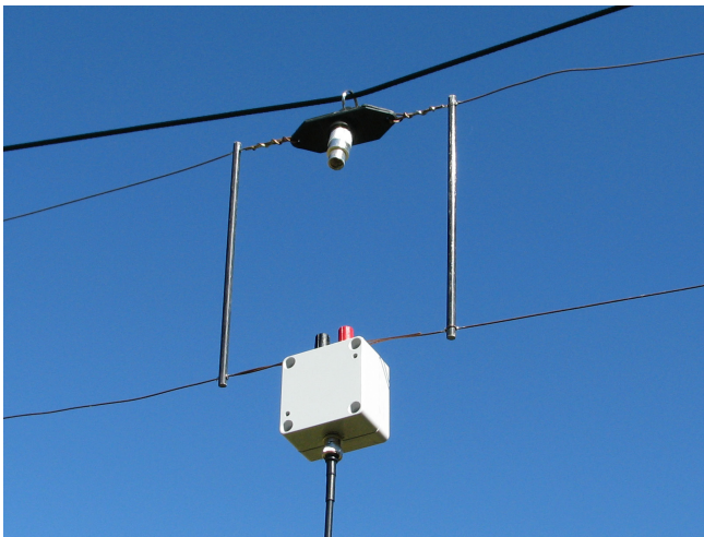
Figure 4 – Center of TFD element. View looking north. Note that the positive (red) terminal is on the east side. This could also be looking east with the positive (red) terminal on the south side.
