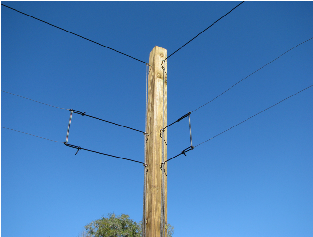
Figure 3 – Top of mast showing screw eyes for halyards and center support rope.
